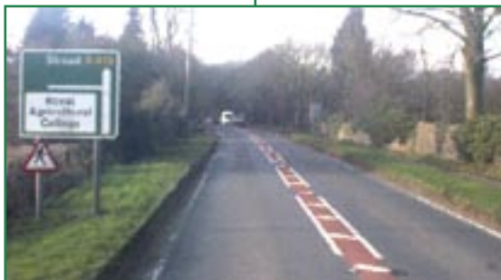
A419 Cirencester to M5 J13 westbound. Improved median score (to be incorporated in later RPS versions) – central hatching
