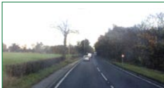
A617. From the A614 to Newark eastbound. 50 mph limit, some 30 mph. High percentage of hedge, then 10m clear zone, some significant trees
