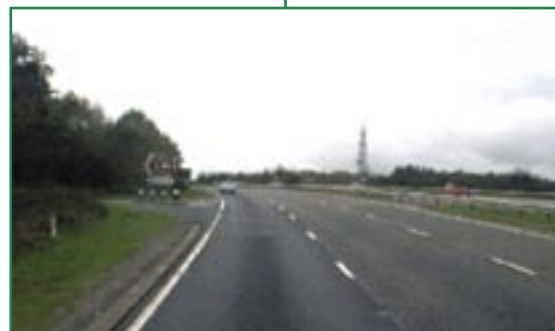
A38 Exeter to Saltash, poor junction score due to short deceleration and acceleration lanes
