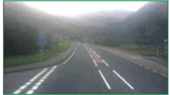
A82 Fort William to Ballachulish. Short section of dual, some 40 mph, short sections of hatching
