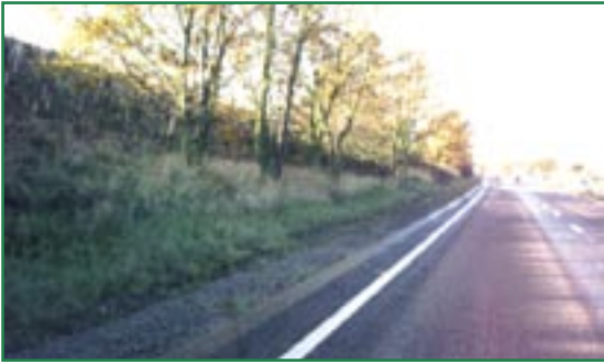
A12 Colchester to Ipswich southbound. Tree line close to edge of dual carriageway
