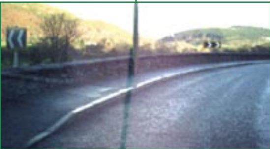
A5 A494 to Llangollen eastbound. Poor run-off score, stone wall as highway barrier, large trees and telegraph poles on apex of bend
