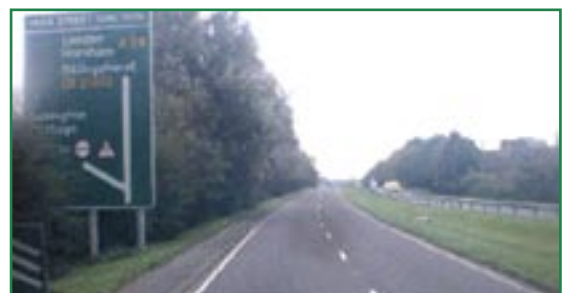
A24 Horsham to A272 northbound. Tree line and very large sign not protected by safety fencing
