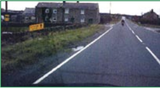
A59 Skipton to Harrogate eastbound. Poor junction score: staggered cross roads without turning lanes
