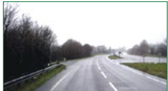
A40 Carmarthen to St. Clears. Poor junction score, at-grade right turn on dual and no acceleration and deceleration lanes
