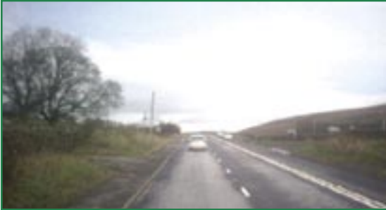
A59. Poor junction score, T junction without turning lane, risk of stationary traffic in outside lane of crawler lane section
