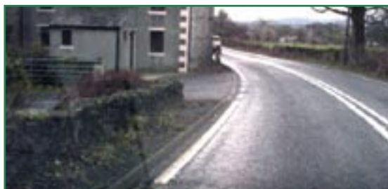
A682. Edge of building very close to edge of road
