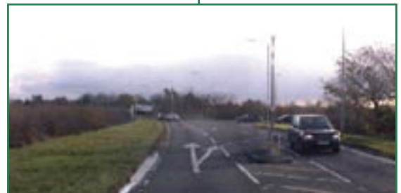
A617. A614 to Newark eastbound. Some protected turning lanes and traffic signals
