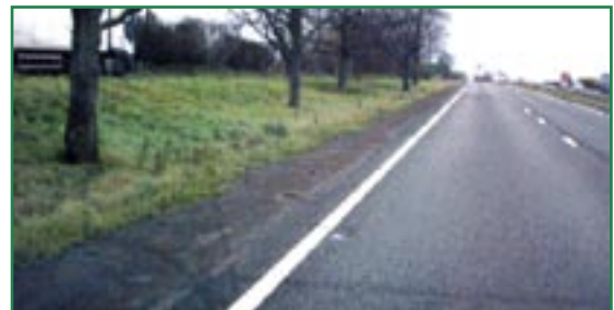
A1 Scotch Corner to Dishforth southbound. Tree line close to edge of dual carriageway. (There was a recent fatal crash on this section of road due to a car hitting tree at side of road.)
