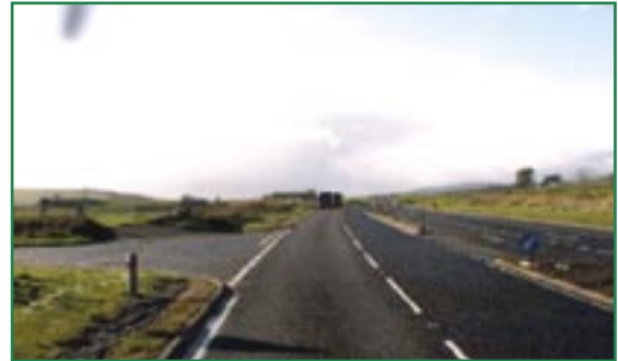
A90 Aberdeen to Perth southbound. Poor junction score, at-grade right turn on dual carriageway and no acceleration and deceleration lanes
