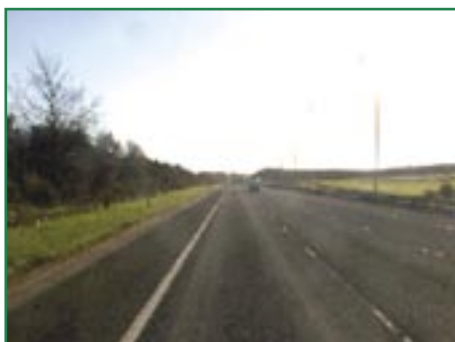
A1M Southbound J15–J14. Poor side score due to tree line
